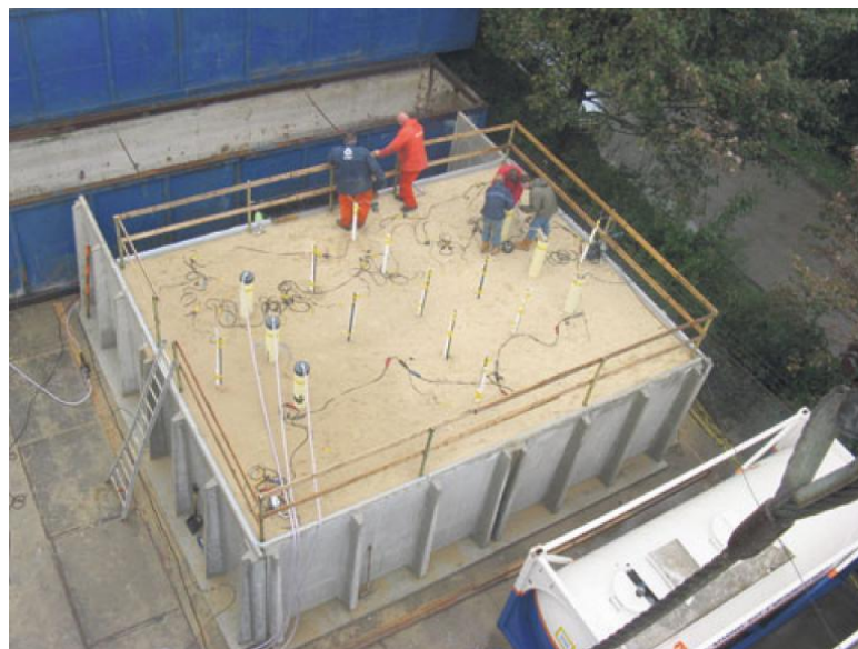
Fig. 9. An application of bio-grouting a soil mass by using cementing bacteria
