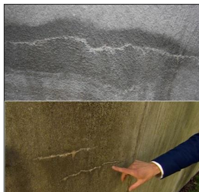
Fig. 12. Self-healing (of cracks) concrete.
